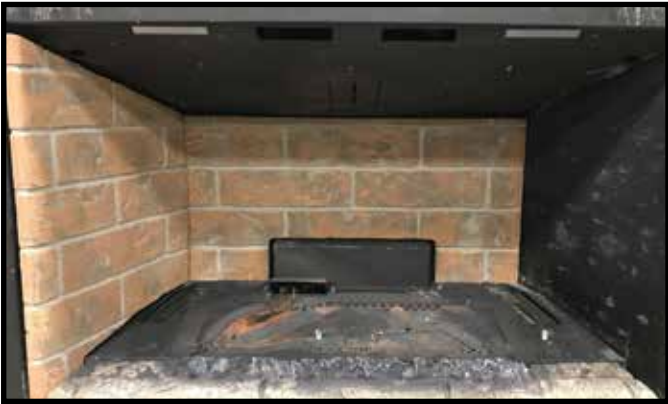
Figure 5 Left Refractory Installed
