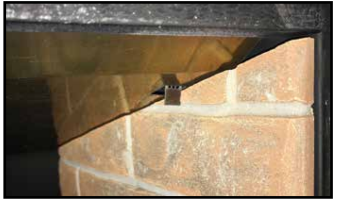
Figure 7 Right Refractory Handbend Tab
