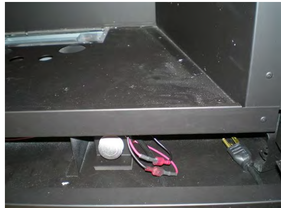
4. Route wires under Firebox to right side of Fireplace.
