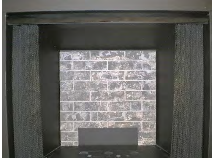
Step Two: Place Back Liner against back wall of firebox.
