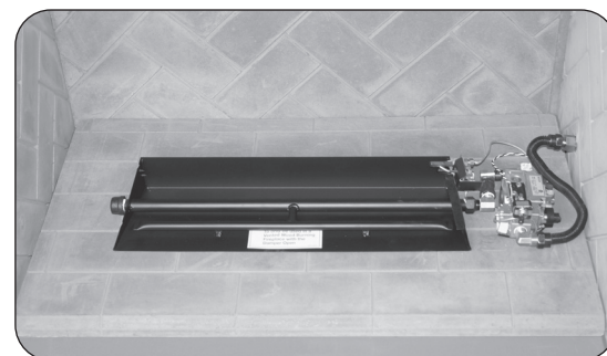
Fig. 15-2 Center burner in fireplace
