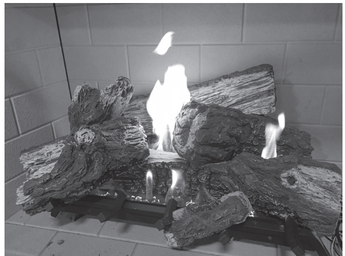
Figure 5.13 - Correct Appearance of Rear Flames
