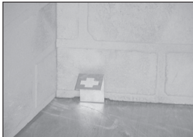
Figure 8.8 Grate Retaining Bracket in Place
