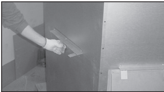
Figure 3.7 Bend Refractory Brackets Back Down
