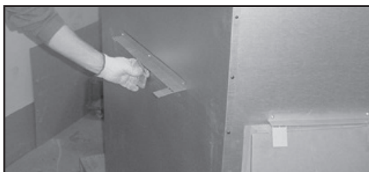
Figure 3.7 Bending Refractory Shipping Tabs Back Down
