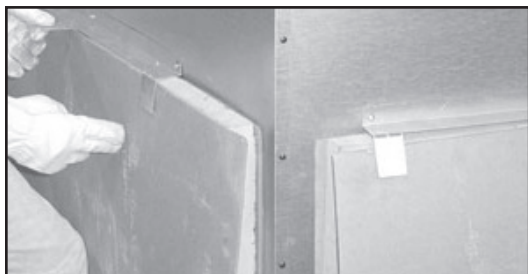
Figure 3.6 Unpacking Back Refractory
