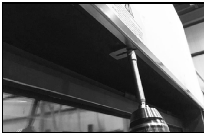
Figure 10.5. Install Trim Ring
